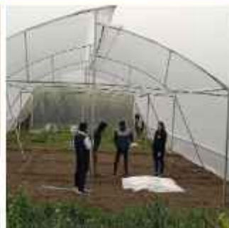
CONSTRUCTION OF POLYHOUSES
