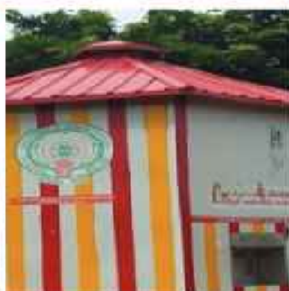
CONSTRUCTION OF R.O. PLANT IN PADMARAKA VILLAGE
