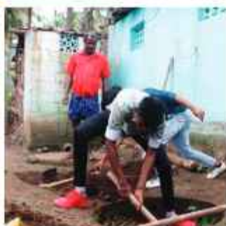
RENOVATION OF TOILETS IN PUTHUPATHI TRIBAL VILLAGE
