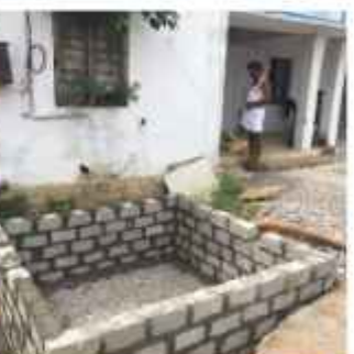
RAIN WATER HARVESTING PITS
